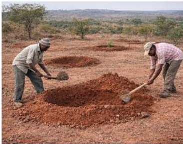
4. Build embankment downslope
