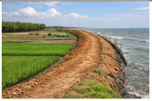
Figure 2.1.29. Seawater control bund constructed along coastal farmland to prevent tidal intrusion.
