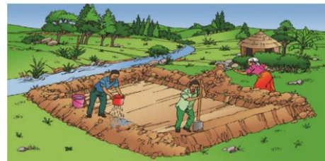
Figures 2.5.7. Excavation, compaction, bund formation, and structural protection
