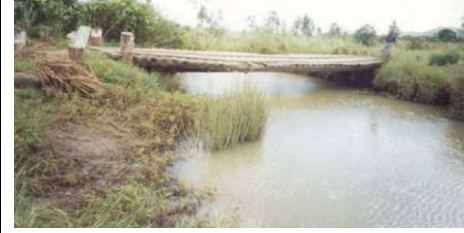
Figure 2.4.17. Community-built timber log footbridge (example of simple crossing)
