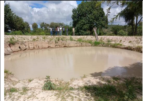
Figure 2.2.7. Completed earth-lined surface water harvesting pond.
