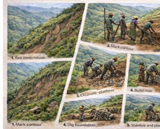
Figure 2.1.25. Stepwise construction of hillside terraces on a steep slope showing contour alignment, narrow cut-and-fill formation, stone riser construction, and vegetative stabilization.
