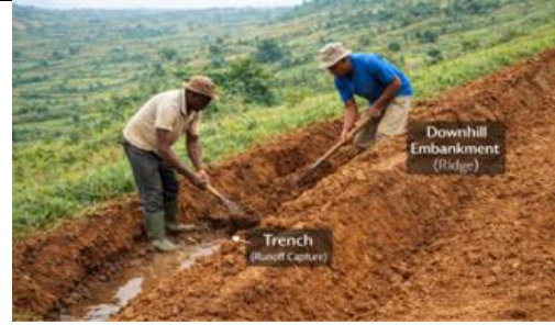
Figure 2.1.13. Cross-section of a Level Fanya Chini Bund showing the upper-side trench and downhill embankment
