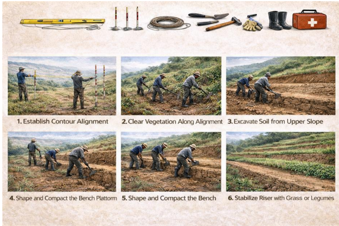
Figure 2.1.22. Step-by-step construction of a bench terrace.
