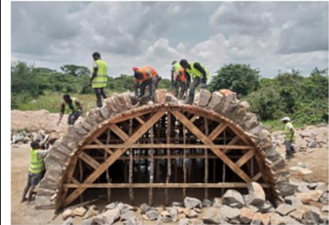
Figure 2.4.18. Ongoing construction of an arch bridge
