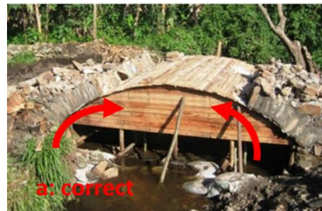
Figure 2.4.24. Keystone placement completing the arch
