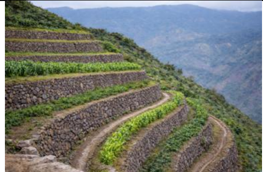
Figure 2.1.23. Hillside terraces showing contour alignment, stone riser stabilization, and terrace platform.
