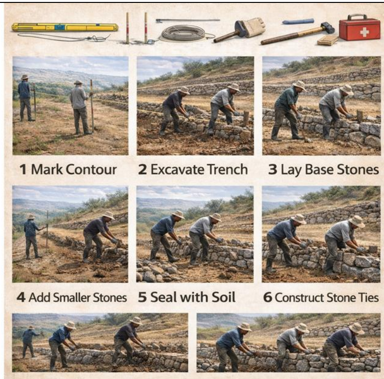
Figure 2.1.18. Step-by-step construction of a stone bund
