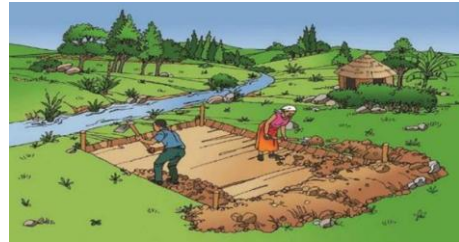
Figure 2.5.6. Excavation and levelling of the check dam foundation area, showing clearance of soil and preparation of a uniform base along the pegged layout.
