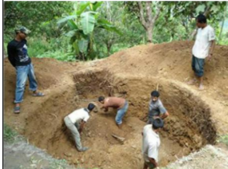
Figure: 2.7.15. Excavation of pit for installation of household biogas digester.
