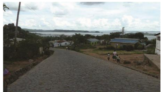
Figure 2.4.2. Typical community stone road constructed under CSPW using locally available materials
