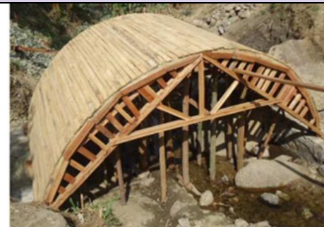
Figure 2.4.23. Prefabricated wooden centring for arch construction.
