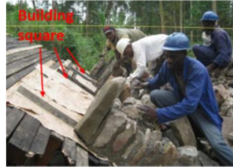
Figure 2.4.25. Alignment control during stone placement
