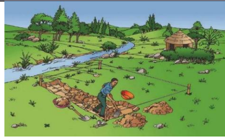
Figure 2.5.5. Excavation and setting out of the check dam foundation using pegged guidelines, with initial placement of stones along the marked trench
