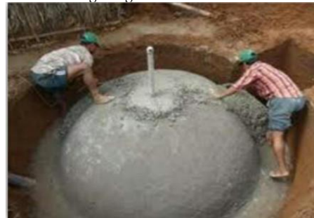
Figure 2.7.16. Construction of the dome-shaped digestion chamber during installation.
