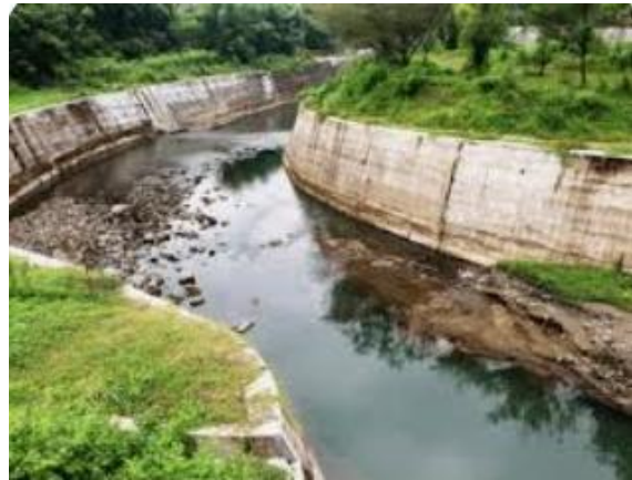
Figure 2.1.66. River retaining using concrete wall.
