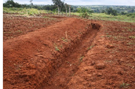
Figure 2.1.5. Cross-section of a Level fanya juu bund showing the embankment and trench orientation.
