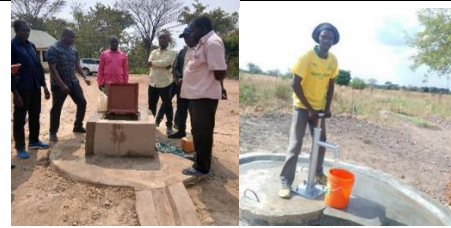
Figure 2.2.4. Examples of community-managed water points, including a protected shallow well with a concrete cover and inspection chamber (a), and a hand pump installed on a lined well for safe groundwater abstraction (b).
