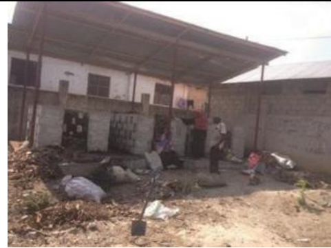
Figure 2.6.7. Urban composting sheds are constructed with concrete block chambers and iron roofing for controlled organic waste management
