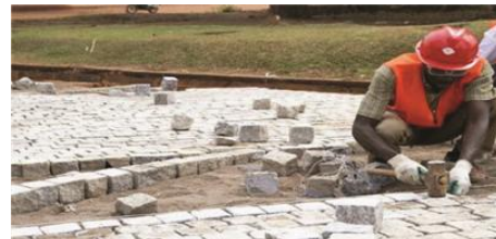
Figure 2.4.9. Community workers aligning and compacting stone surface under CSPW
