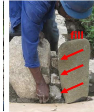
Figure 2.4.26. Filling of gaps between arch stones
